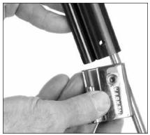
Slip feeder into place and firmly push upwards.
