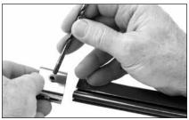
**Tip:** Trim cap holes are different diameters. Make sure 3/16" (5 mm) drill bit fits through hole and foil side grooves face up.
